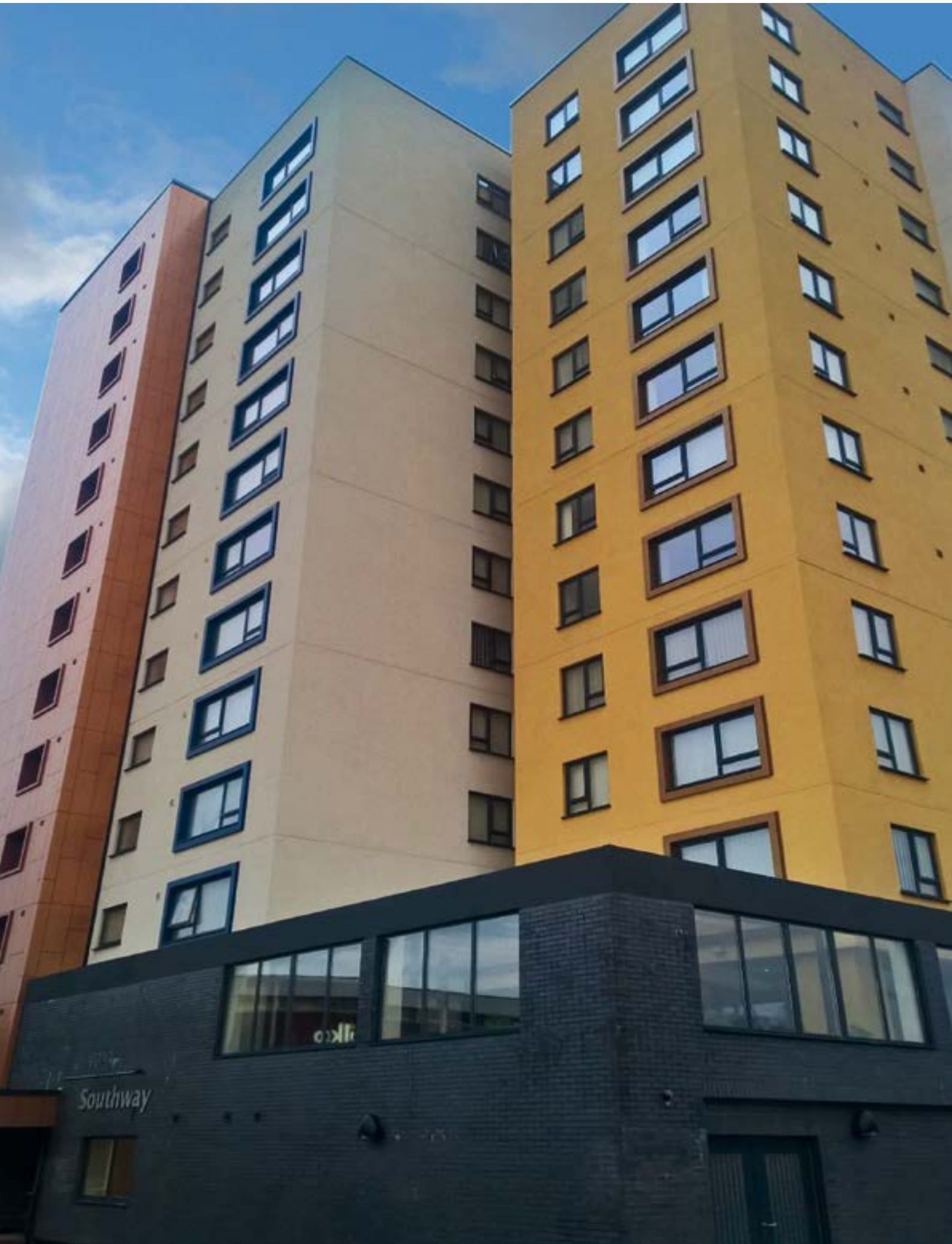
Southway Tower, termok8® fenolico, Manchester, UK
