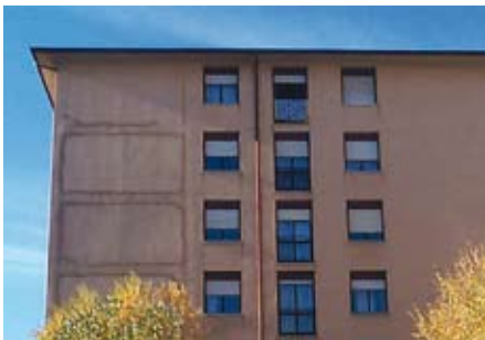
Cracks in the curtain wall: insulation on the inside excludes the outer walls from the "building system" abandoning them to their own thermal destiny
